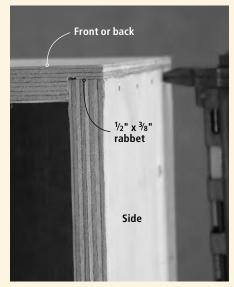
Joining drawer sides to the front and back can be as simple as cutting a rabbet. Then you can use glue and nails to complete the joint.
