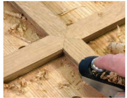
**Payday.** Flush the surfaces of the completed joints with a sharp block plane, and take a moment to feel proud. Then get back to work; there are a bunch of these.
