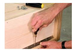
When installing a piano hinge, first install just a few of the screws. Then test the hinge.
