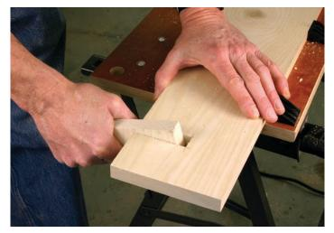
Test fit each joint as you go by fitting a piece of scrap wood. Take note of where the joints are too loose or too tight and correct your technique when you cut the next joint. Don't worry if the first joints have some gaps. The project will still come together if you're not perfect. The idea is to practice and get better with each attempt.
