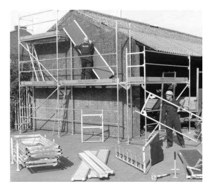
Fig. 10.17 Frame system scaffold
