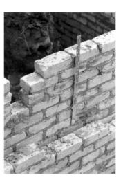
**Fig. 5.9** *Positioning holding- down straps*
