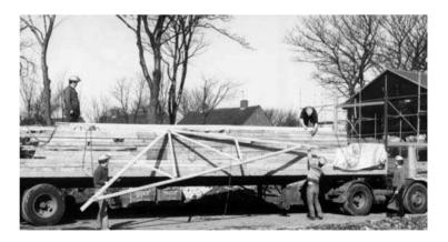
Fig. 8.23 Unloading trussed rafters
