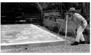
**a** First sighting through lower telescope – using the fine traverse adjusting screen to bring the 'cross-hairs' in line with the front edge of the concrete raft (slab)
