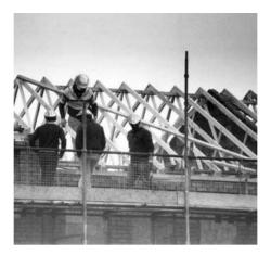
Fig. 8.28 Trussed-rafter roof being erected
