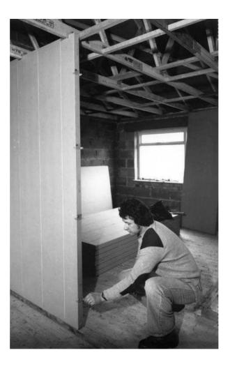
**Fig. 9.14** Installing a 'Karphos' partitioning system
