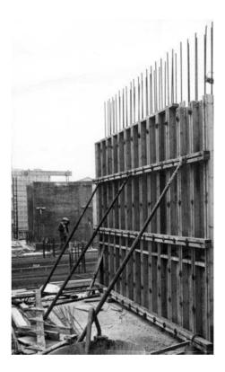
Fig. 3.13 Erection of wall form
