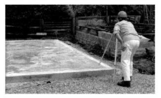
**b** Sighting through the upper telescope to ensure that the side edge of the concrete raft is at a right angle (90°) to the front
